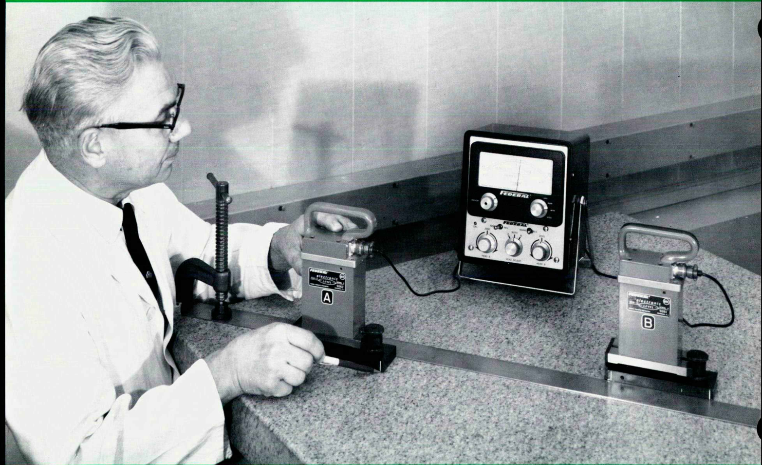
The Differential Electronic Level is being used here to profile a surface plate. Input from the two heads is received in opposite modes, so that the Amplifier will respond only to changes which affect them differently. Consequently, any tilting of the surface plate as it is being profiled is ignored.
